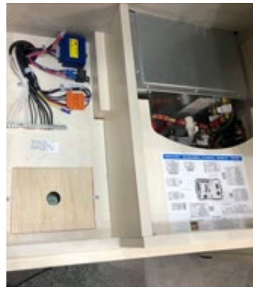
50 AMP BATTERY DISCONNECT BREAKER
