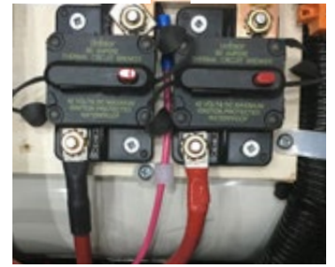
50 AMP BATTERY DISCONNECT BREAKER
