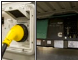
Shore Power or Generator
