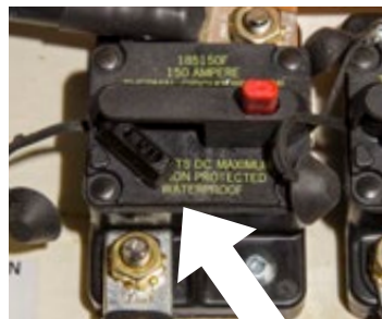
ARM DOWN INDICATES TRIPPED BREAKER
