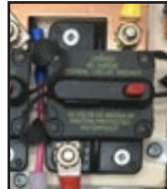
80 Amp Charger Output Breaker
