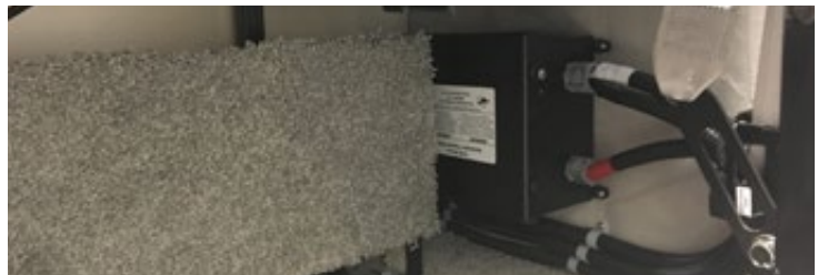
ARM DOWN INDICATES TRIPPED BREAKER
