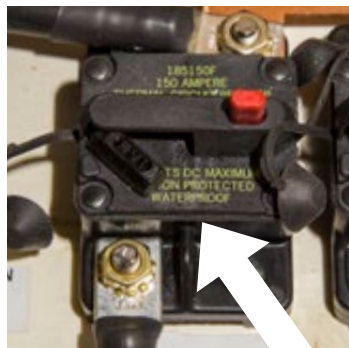
ARM DOWN INDICATES TRIPPED BREAKER
