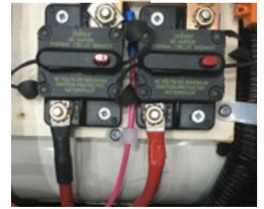
50 AMP BATTERY DISCONNECT BREAKER
