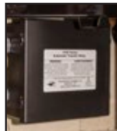
Automatic Transfer Switch
