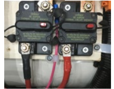
50 AMP BATTERY DISCONNECT BREAKER
