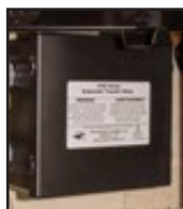
Automatic Transfer Switch
