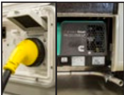
Shore Power or Generator
