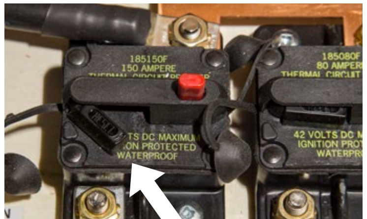
ARM DOWN INDICATES TRIPPED BREAKER
