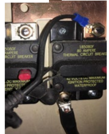
80 AMP BATTERY DISCONNECT BREAKER 80 AMP GENERATOR BREAKER
